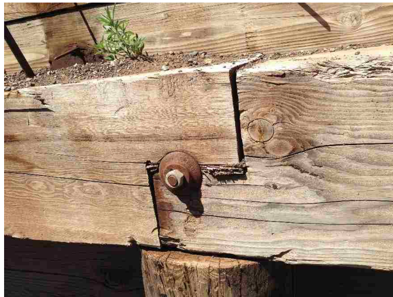
Figure 3-11: The Joined Girder of Timber Bridge
