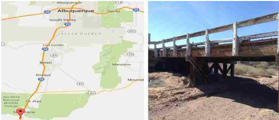
Figure 3-16: Location and Street View of Bridge #1676
